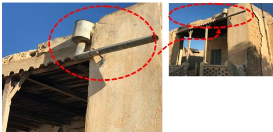
Figure (16) Rain drainage systems as a very important source for storing water. Source: Field visit of the researcher,2025
