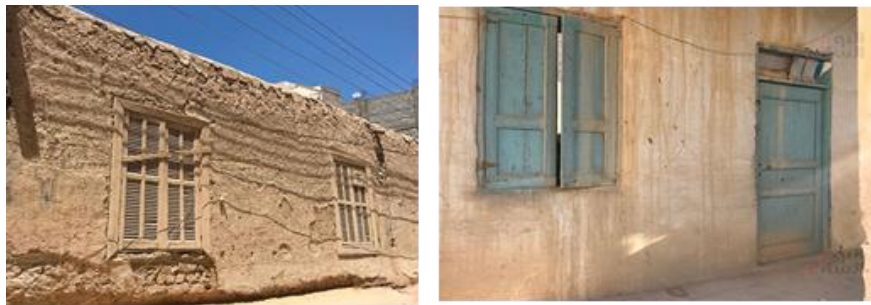
Figure (13) wooden windows made of shutters with large size on the outside of the house Source: Field visit of the researcher,2025
