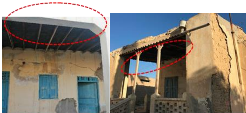
Figure (10) Wooden ceilings on roof the veranda area in Al-Arish house Source: Field visit of the researcher,2025
