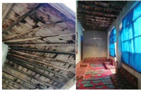
Figure (9) Wooden ceilings on corridors between the rooms in Al-Arish house Source: Field visit of the researcher,2025
