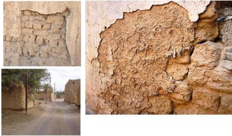
Figure (12) Using local clay and mixing it with barley straw to maintain thermal comfort inside the houses.
