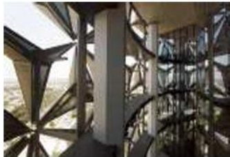
Fig. 23. Illustrates the effect of the external shell on the internal ventilation of the building [17].
