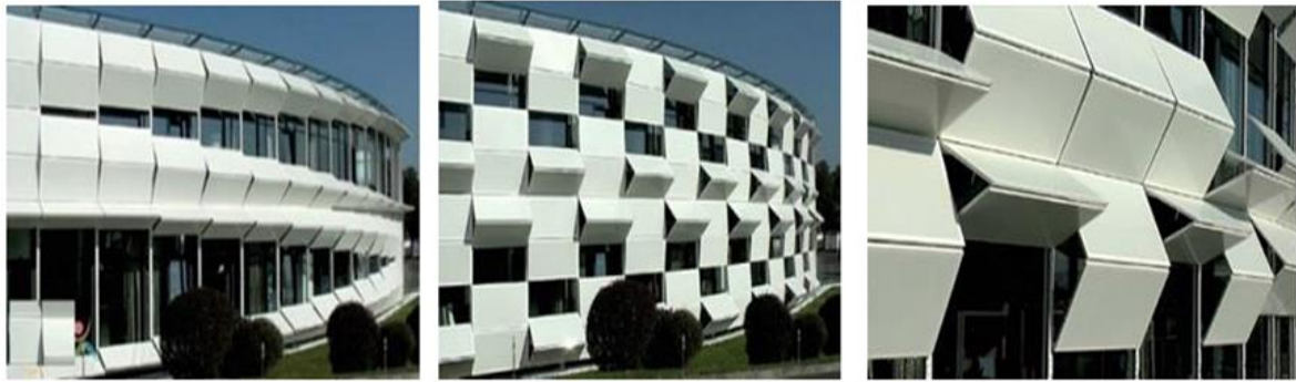
Fig. 15. The shape of the facade changes as the units open and close and interact with climatic conditions [8].
