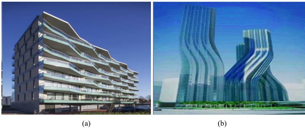
Fig. 3. Refers to examples of buildings that demonstrate optical illusions by curving vertical and horizontal lines to make the facade look like it's dancing [8].
