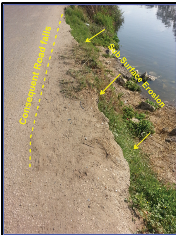
Figure 4. The asphaltic road partially falls on the southwestern shoulder of the submerged Syphon's body.
