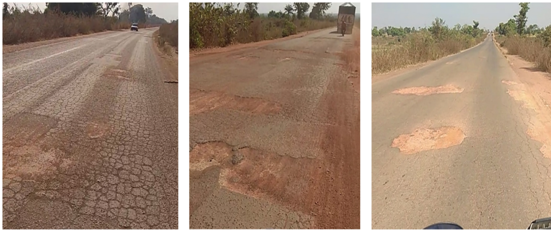
Figure 2. Some sections of the Lafia-Shendam Road showing cracks and potholes on the road pavement.
