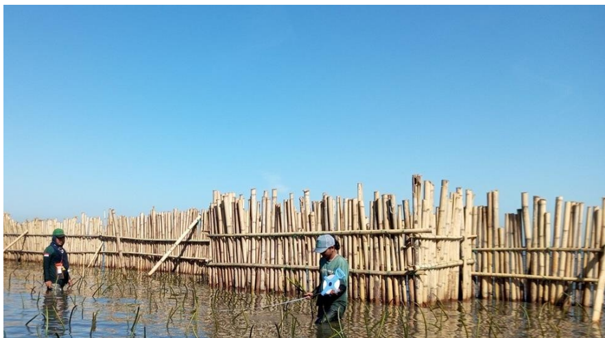
Fig. 3. A bamboo-based wave breaker (Seawall)
