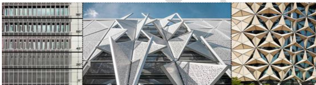
Fig. 6: The use of moving systems on facades is shown to be beneficial in shading within spaces. (Enrich Ruiz-Geli, Media-ICT, www.worldbuildingsdirectory.com/project.cfm?id=3752 , (Accessed: 7, 2025).
