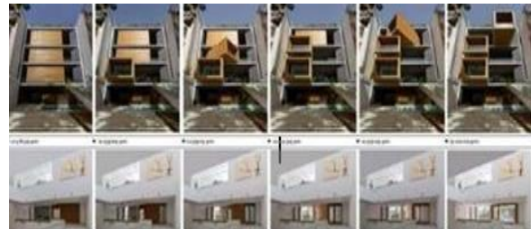
Fig. 5: Shows the reorientation of rooms in the Sharifi-Ha house according to the climatic seasons. ( https://www.archdaily.com/522344/sharifi-ha-house-nextoffice , access 7-2025)
