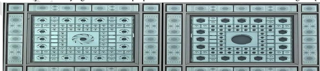
Fig. 7: Modules of the south façade of the Arab World Institute show the kinetic façade to achieving ventilation, ( https://charifbo.medium.com/exploring-kinetic-architecture , and access 8-2025).
