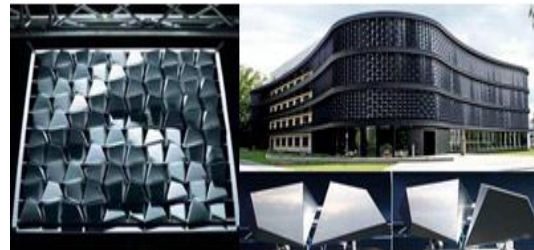
Fig. 10: Automatic window opening control based on users' lighting need The Flare-fagade system is a modular dynamic system that can be installed on building's facades or any wall surface. ( https://www.academia.edu/ , access 7-2025.)
