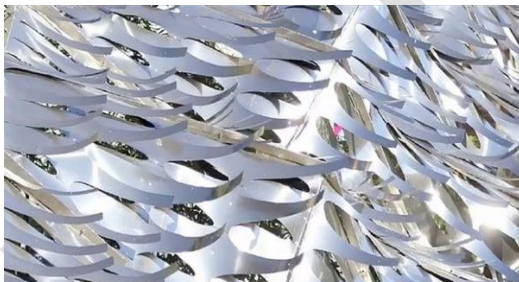
Fig. 3: Thermal Bimetals [Spendlove, T. (2016). Breathing BioMetal Regulates Building, erging-materials-thermo-bimetals Temperature - A Moonshot Project > ENGINEERING.com. [Online] Engineering.com. Available at: http://www.engineering.com/DesignerEdge.access 7-2025].
