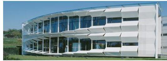
Fig. 9: Automatic window opening control based on users' lighting needs. ( https://alubuild.com/en/architecture-kinetic-facades/ access 8-2025)
