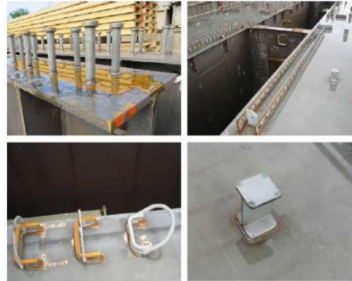
Figure 2. Typical Shear Connectors
