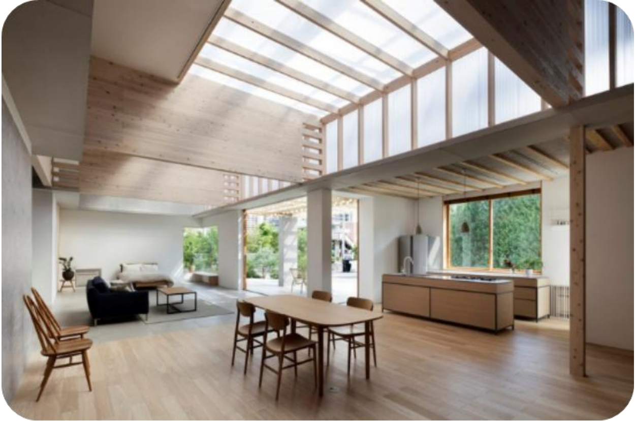
Figure 5. Demonstrates the use of transparent or semi-transparent polycarbonate as a roofing and window covering, along with appropriately placed openings. This provides soft natural lighting, reduces reliance on artificial lighting, and allows for sustainable natural ventilation to maintain indoor air quality (URL: https://shorturl.at/f6E0e )
