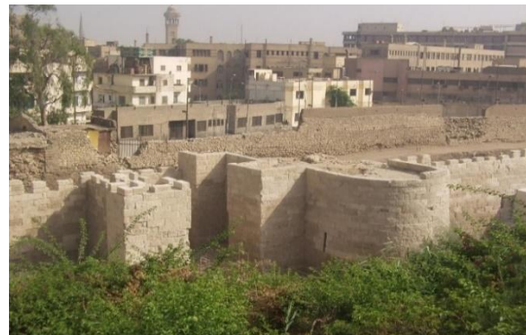
Fig. 14: the wall after restoration
