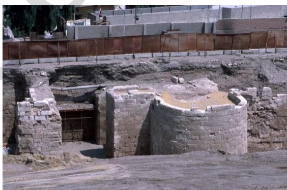
Fig. 13: loss of stone details before restoration
