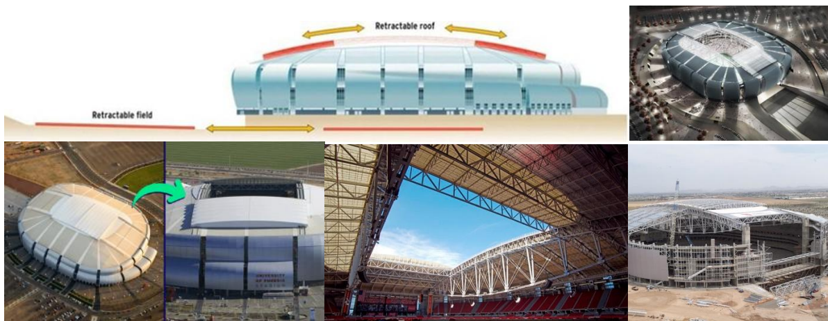
Fig. 9: Illustrates the motion of retractable roof of State Farm Stadium; source: [13]
