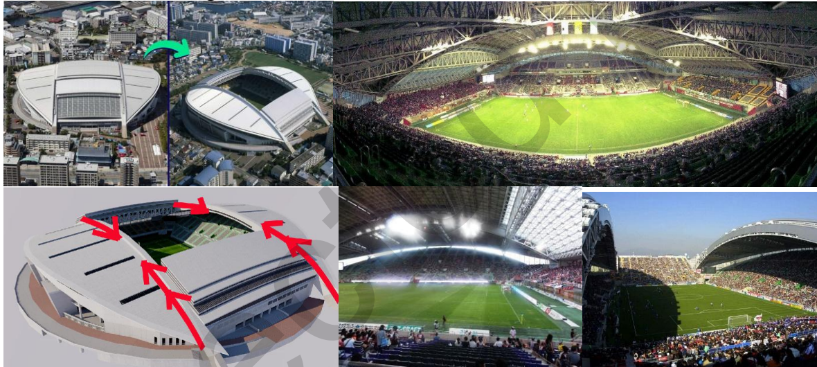
Fig. 8: Illustrates the motion of retractable roof of Noevir Stadium; source: [12]
