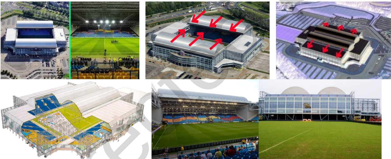
Fig. 6: Illustrates the motion of retractable roof of Gelre-Dome Stadium; source: [10]
