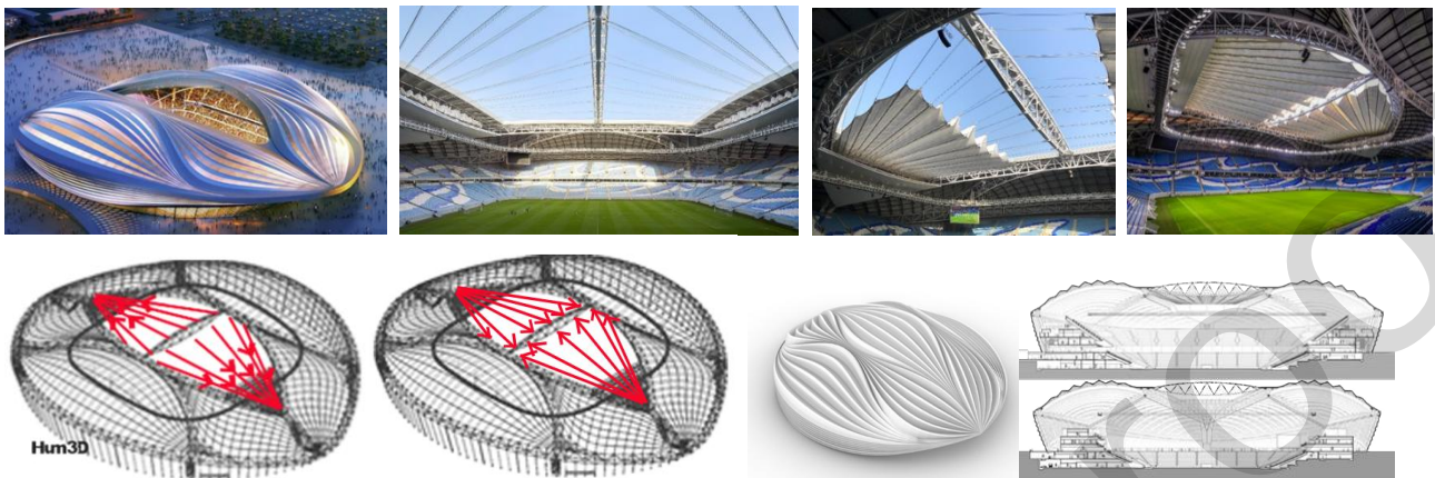
Fig. 13: Illustrates the motion of retractable roof of Al Janoub Stadium; source: [16]
