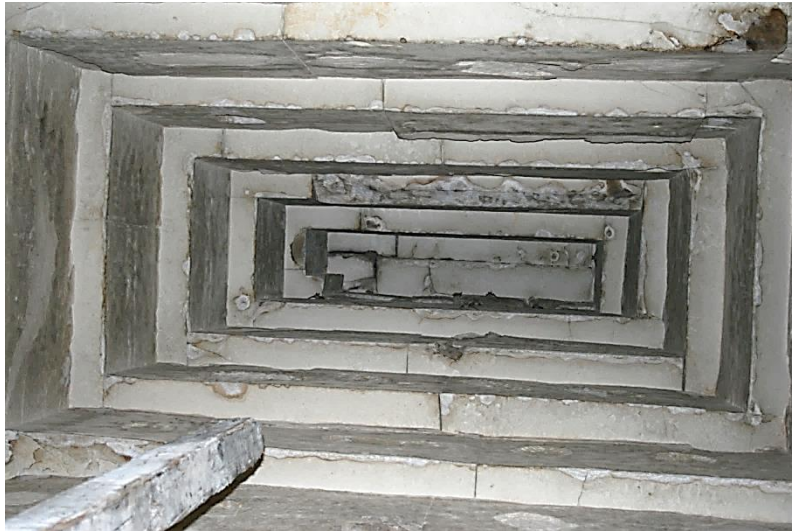
Fig.2. Stepped ceiling inside the bent pyramid of Sneferu (Photo: The author).
