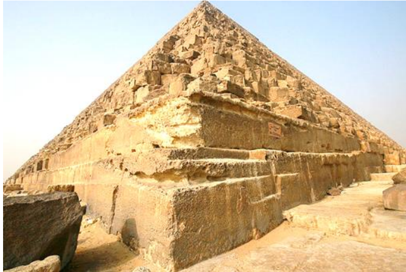
Fig.7. Rock outcrop as part of the pyramid structure of Khufu (Photo: The author).
