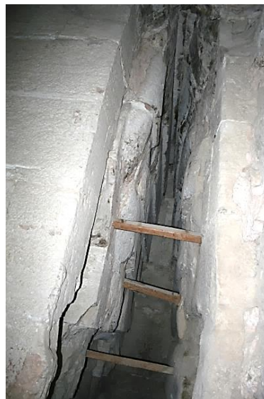
Fig.17. Wooden beams in the burial chamber of the Bent Pyramid (Photo: The author).
