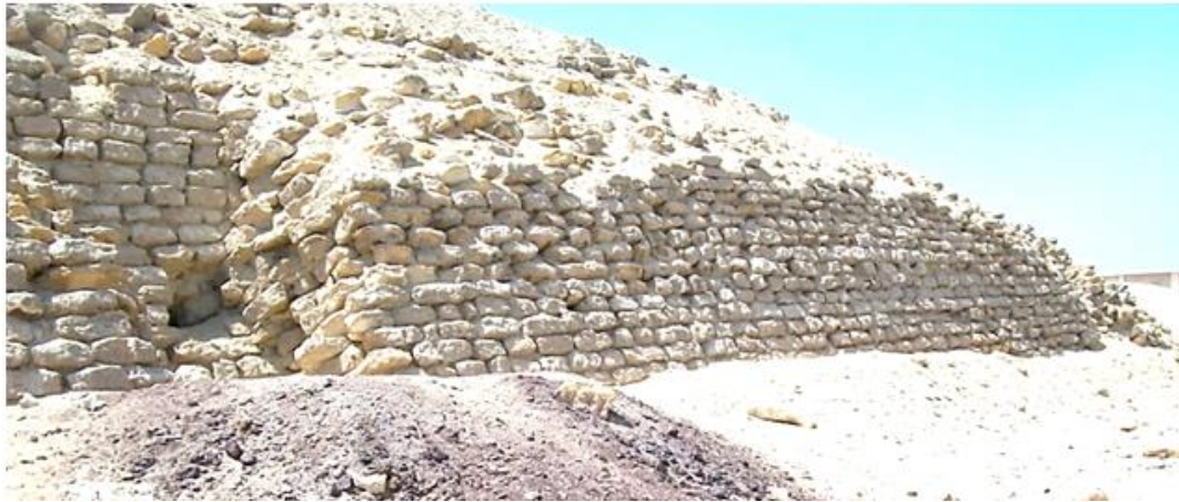
Fig.19. Stones and mortar tilt inward in Khafre's Pyramid (Photo: The author).
