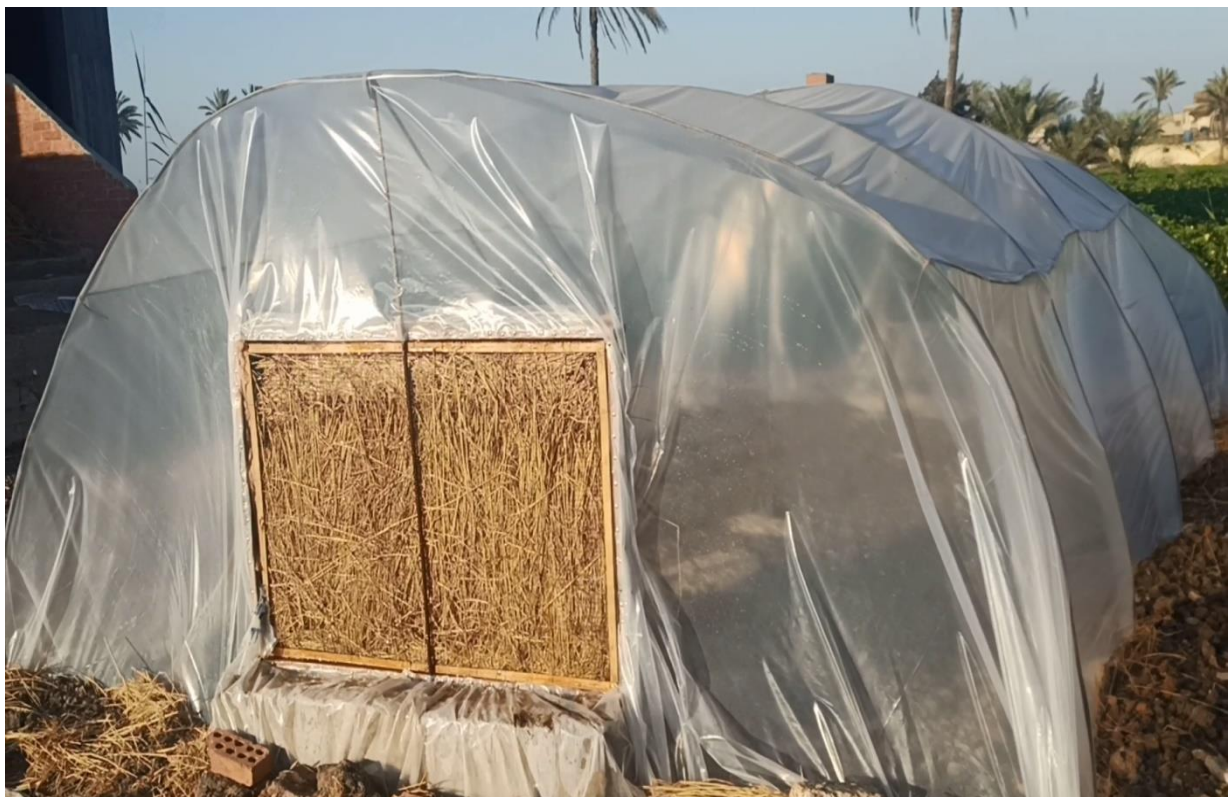
Fig. 4. Rice straw cooling pad is installed in the middle of the northern side of the greenhouse
