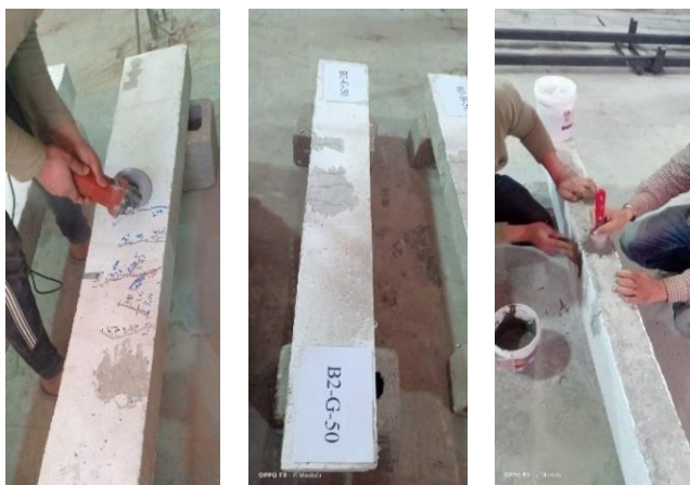
Expanding cracks Cleaning surfaces Filling the cracks
