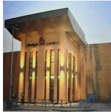
Fig. 12: Mall of Egypt [24]
