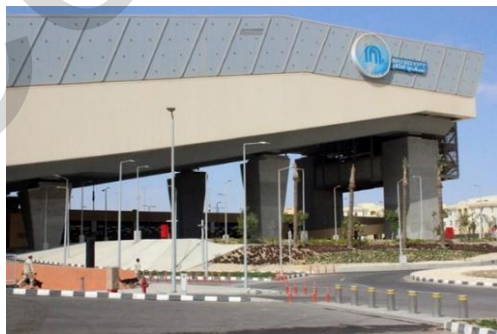
Fig. 15: concrete surfaces responds to temperature [23]
