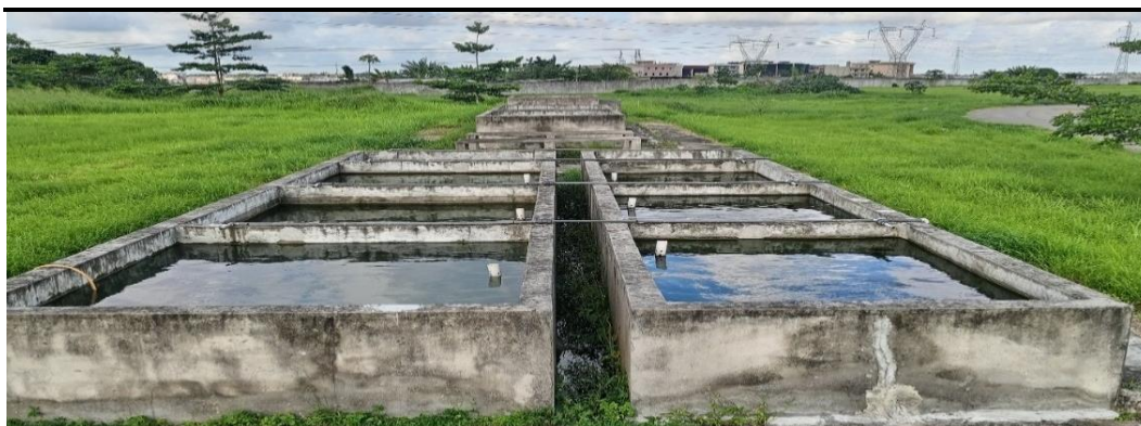
Fig. 1. Experimental structures used for the trials
