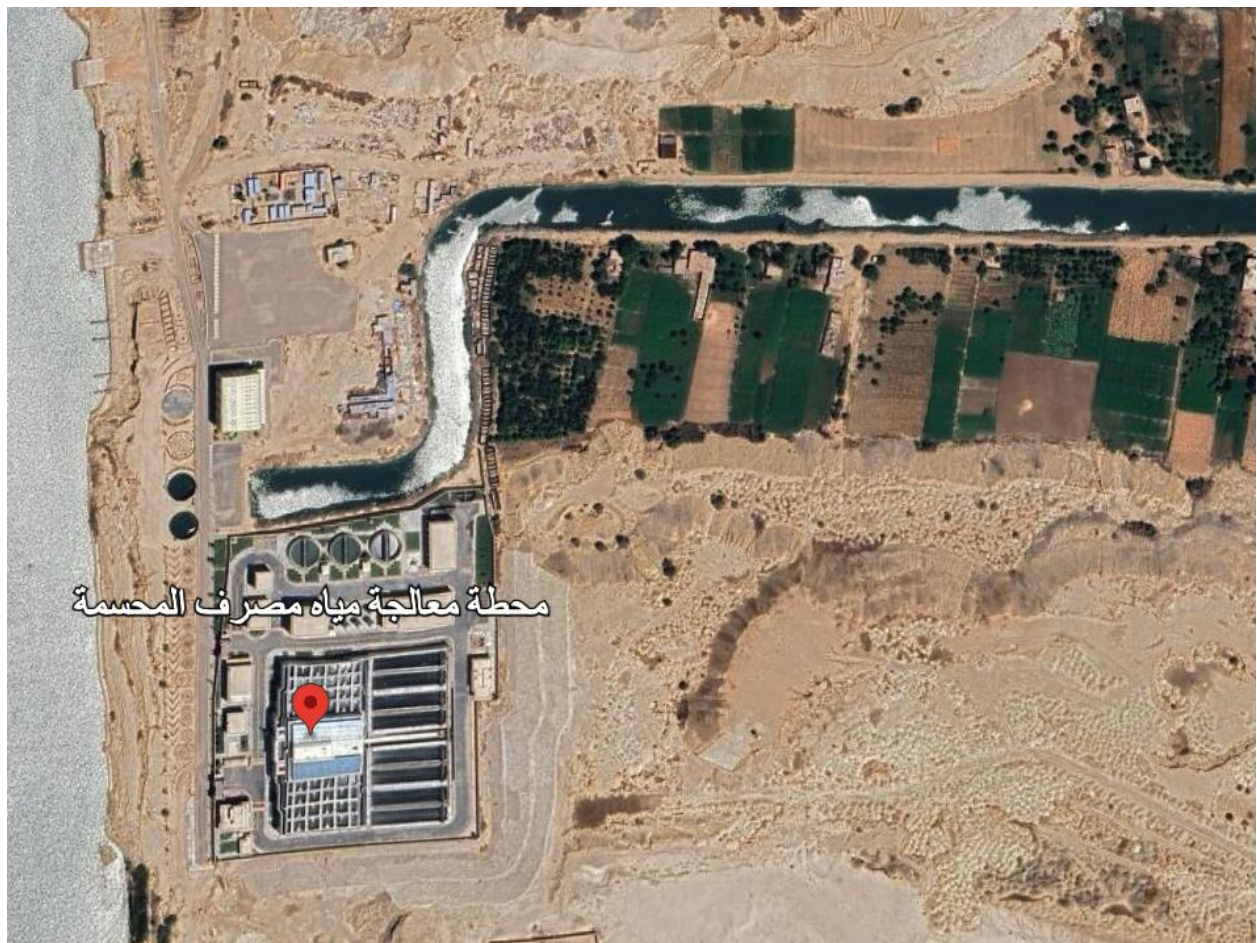
Figure 2. Al-Mahsama (waste water treatment plant) WWTP in the eastern region of the Suez Canal.
