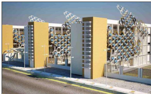
Figure 15: Visualization of the proposed of uniform integration BIPV system.
