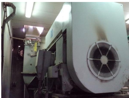
Fig. 2 Photographic image for atomization air blower
