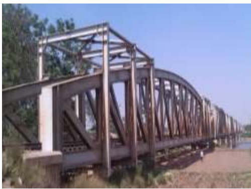
Figure 1: General view for the tested bridge
