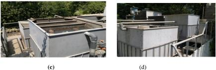
Fig. 2. Degreasing tank followed by settling tank.
