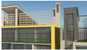
Fig. 36. Micro wind turbines rows installed on the roof, Source: Author
