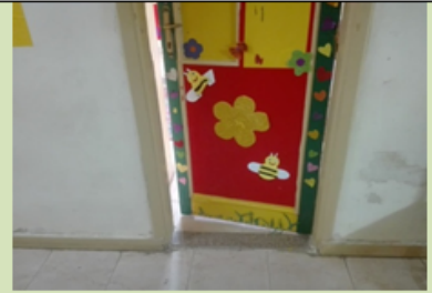
Fig. 20: Field photo of Classroom door.
