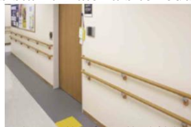
Fig. 11. handrails are installed on the walls, for all children of different ages and abilities. [11]
