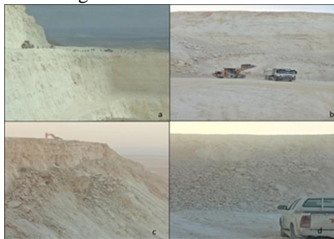
Fig. 6. Blasting trial -3 during charging and muck pile fragmentation
