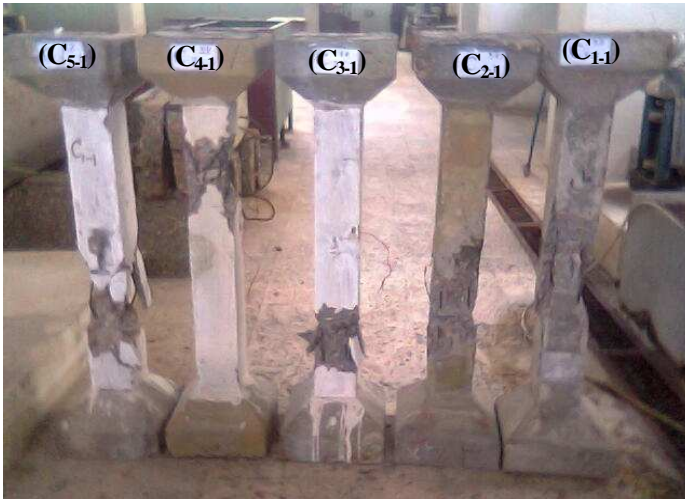
Photo 1: Cracks and mode of failure of R.C. tested columns (Group A)
