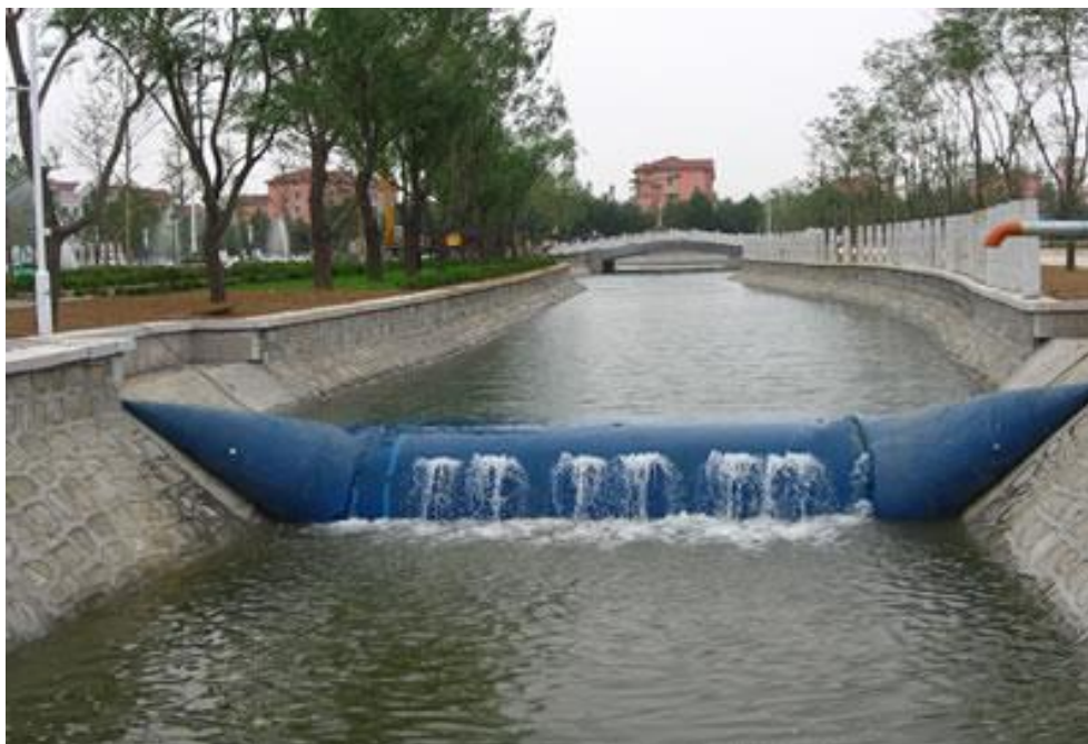
Fig. 12: Using rubber weir to raise U/S water surface level [18]
