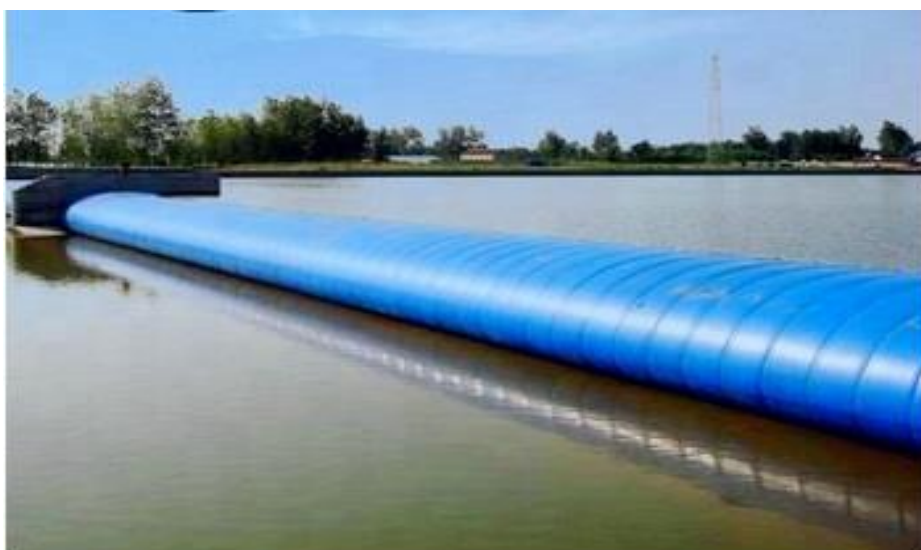
Fig. 11: Application of multiple spans rubber weir in open channel [17]
