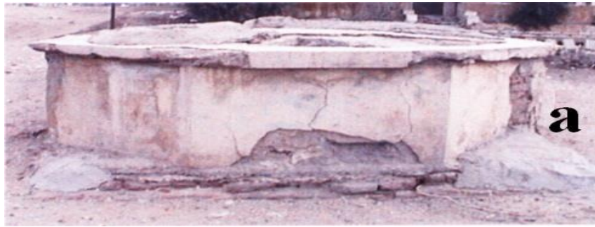
a- The original site with cement building surrounding the spring
