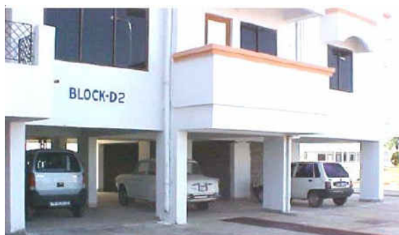
Fig. 1. Typical example of open ground story building[1]
