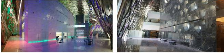
Fig. 31. The spacious interiors show the titanium dome with no internal columns and the reinforced concrete buildings inside. [33].
