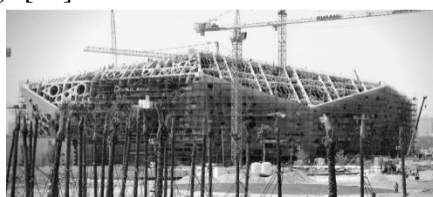
Fig. 14. The structural system for the outer skin [25]
