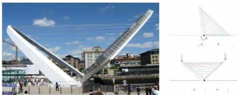
Fig. 4. Gateshead Millennium Bridge, Newcastle [2].
