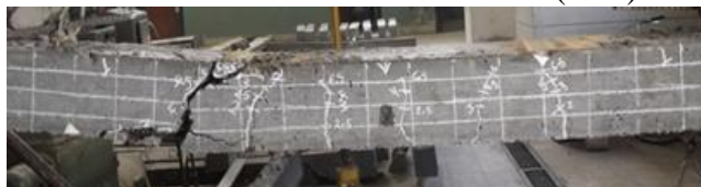
Photo 5. Mode of failure of beam (BFS0).
