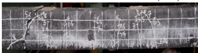
Photo 2. Mode of failure of beam (BF1).
