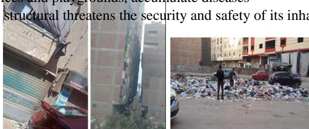
Fig. 9. Garbage accumulation and structural deterioration.(By: researcher, 16-6-2019)
