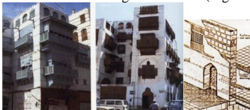
Fig. 13. Different types of Rawashin that cover the outer openings of buildings in the western region to protect them from the sun.
