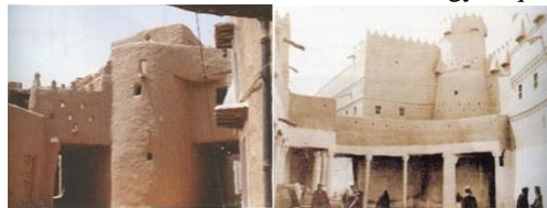
Fig. 8. The narrowness of the external openings of the buildings in the central region achieves thermal comfort inside the building
