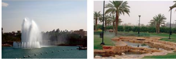
Figs 18 & 19. Pictures for Salam Park, Riyadh, KSA
