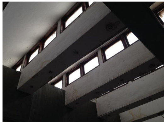
Fig. 5. Sawtooth toplighting technique that is used to enhance daylighting deep into the space (above right) [Researcher].
