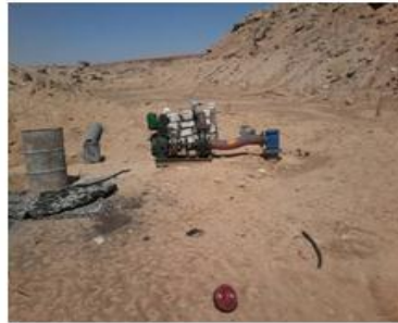
Fig. 9. Drilling of wells in WAPA
