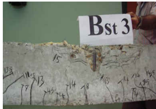
d- Shape of failure of beam (Bst3)
