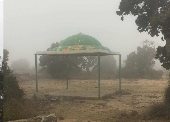
Figure 7: National park shelter
