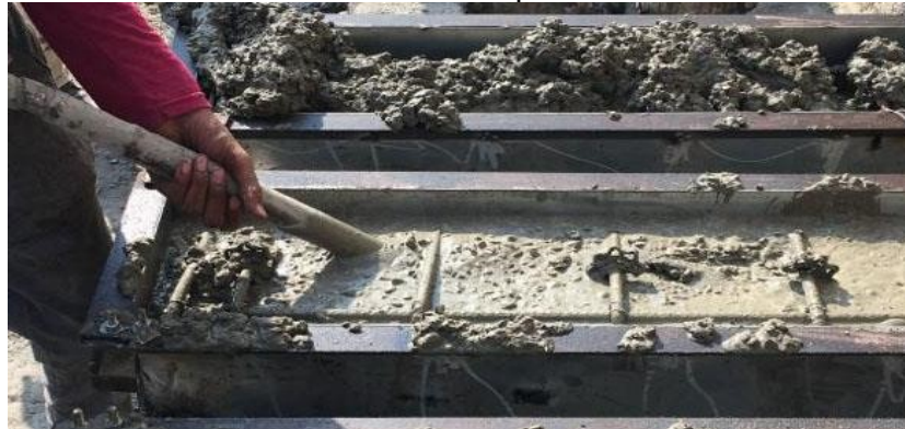
Fig.4 Casting of columns
