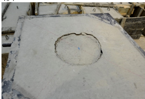
Fig. 12: Punching shear failure of the concrete core
