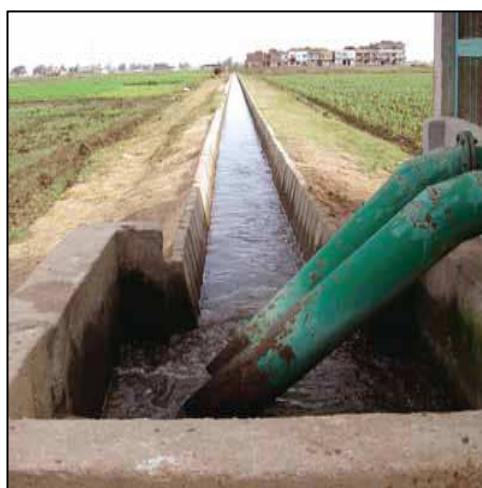
Photo (2) Elevated Mesqa after improvement
