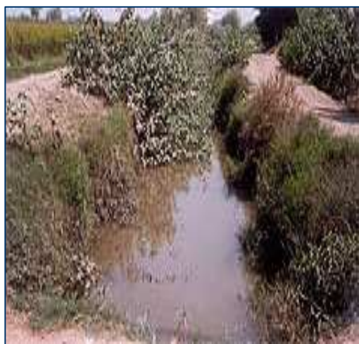
Photo (1) Earthen Mesqa before improvement
