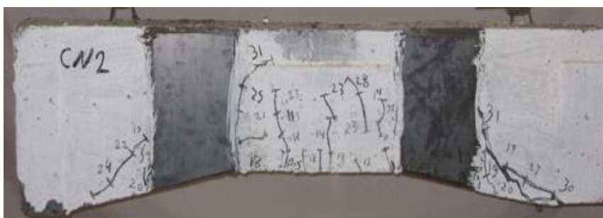
Fig. (4):Crack pattern of beam "CN.2". With thickness of steel plate (2.00 mm)
