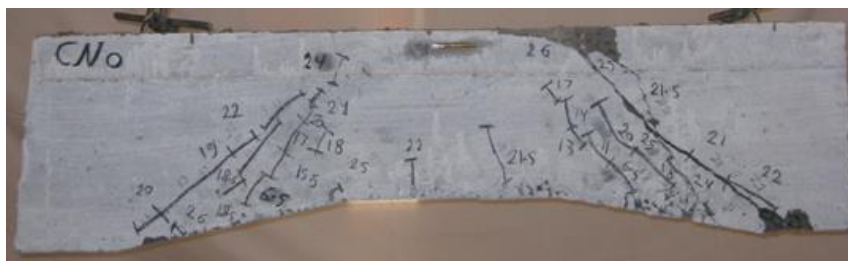
Fig. (2):Crack pattern of beam "CN.0".
