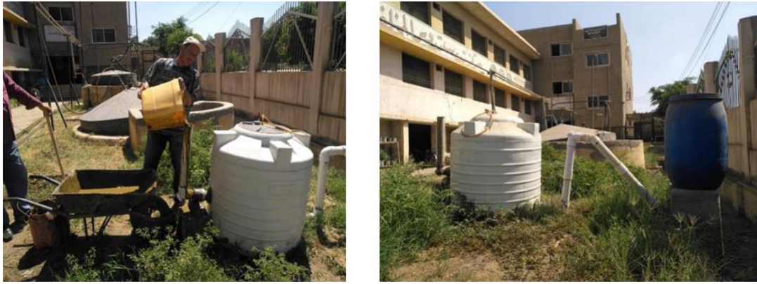
Fig (1): Photo of the biogas unit.
