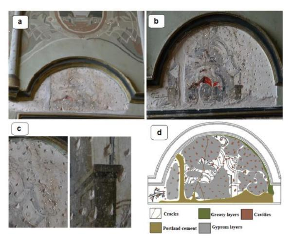
Fig. 1. a) An example of the recent renovations of the National Military Museum 'El Harem palace', uncovered area is also observed, b) A close-up of uncovered area on the walls after preliminary cleaning process, c) Details of the motifs representing the Rococo style, d) Documentation using AutoCAD program reconstruction of the main deterioration aspects affecting the mural.
