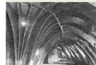
Fig-4 Lofts of the mild house, with the structure of diaphragm arches by Gaudi.
