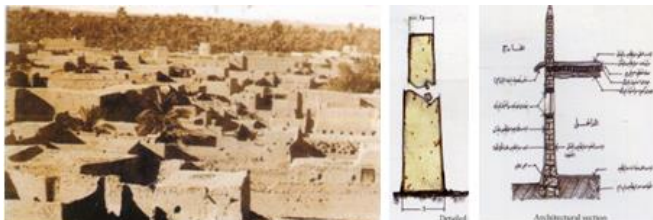
Fig. 22. Mud is the main traditional building material in the central region [11]
