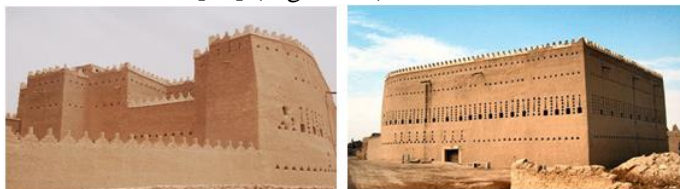
Fig. 21. Small openings in the exterior elevation
