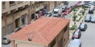
Fig. 19. Electricity room where solar panels will be roof-mounted [4].
