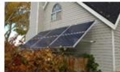
Fig. 20. Wall mounted solar panels, used as shades [16].
