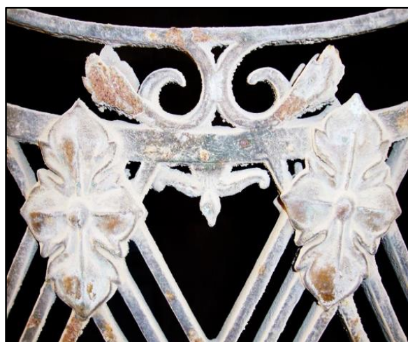
Fig. 2: shows the iron was corroded due to paint detachment.
