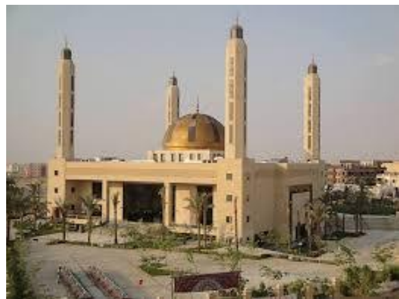
Figure 18 Hassan Sharbatly Mosque new Cairo as an example of an urban center in its location. Source: www.hasfound.org
