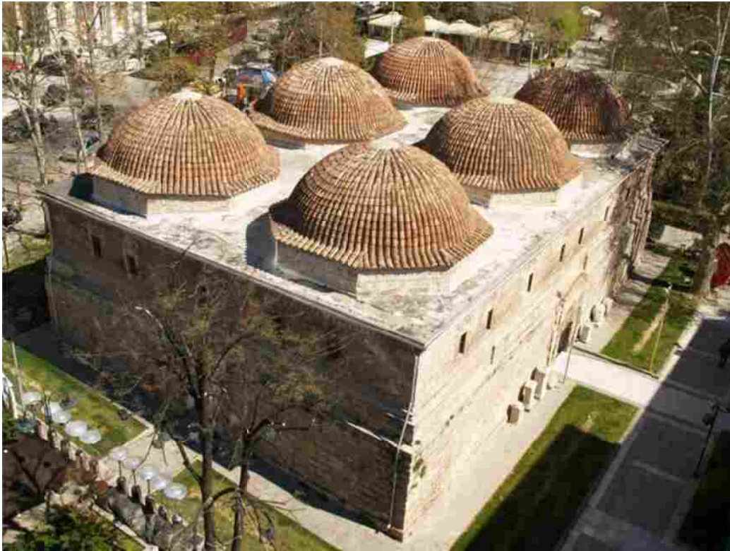
Fig. 7. The Serres Bedesten, Above general view showing the roof and SE and SW facades 41
