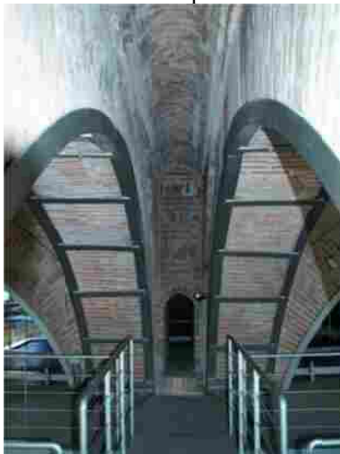
Fig. 19. The Thessaloniki Bedesten, the interior, the double arches and pendentives
