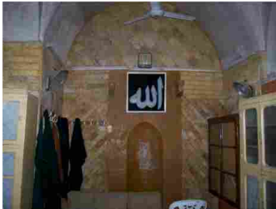
Pl. no.11: The mihrab of the mausoleum. By the author in July 2010.
